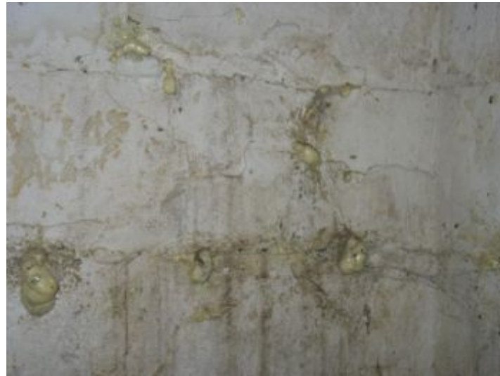
previously repaired small cracks and spalling
