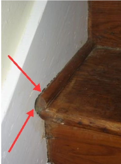
steps are pulling away from the wall
