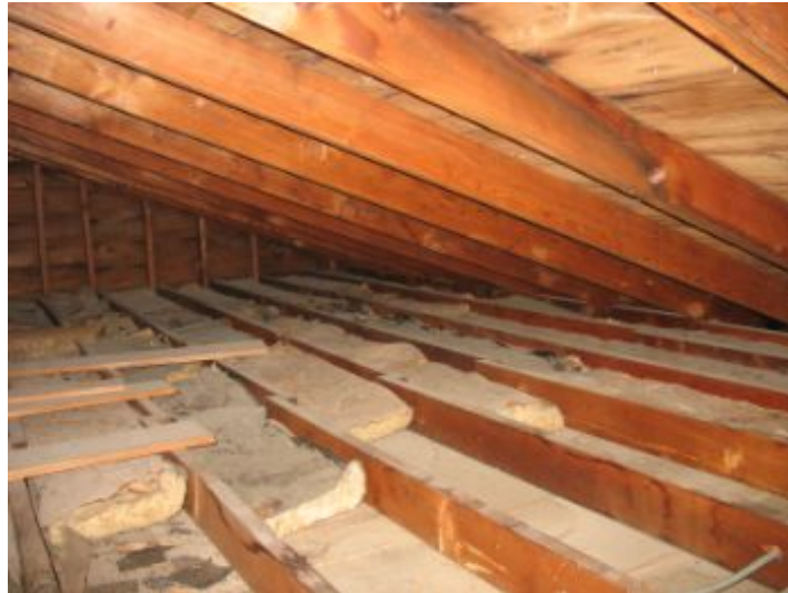
irregular and insufficient installation, many areas have no insulation present.
