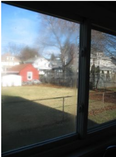
failed sealed, moisture between panes
