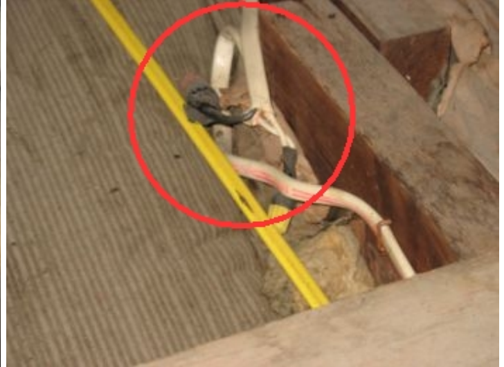
several splice connections made without J-box
