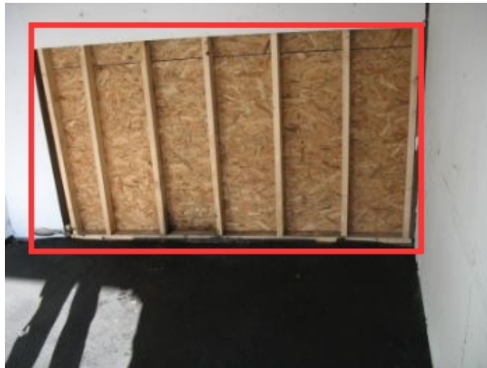
missing drywall in areas
