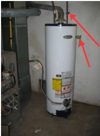
FYI - gas shutoff location - and missing T&P valve extension
