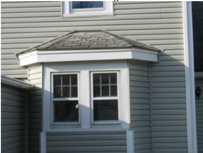
bay window roof needs replacement
