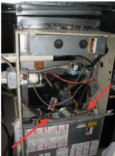
Furnace - some rust present under the condensate fan
