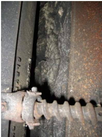
damper tested / checked
