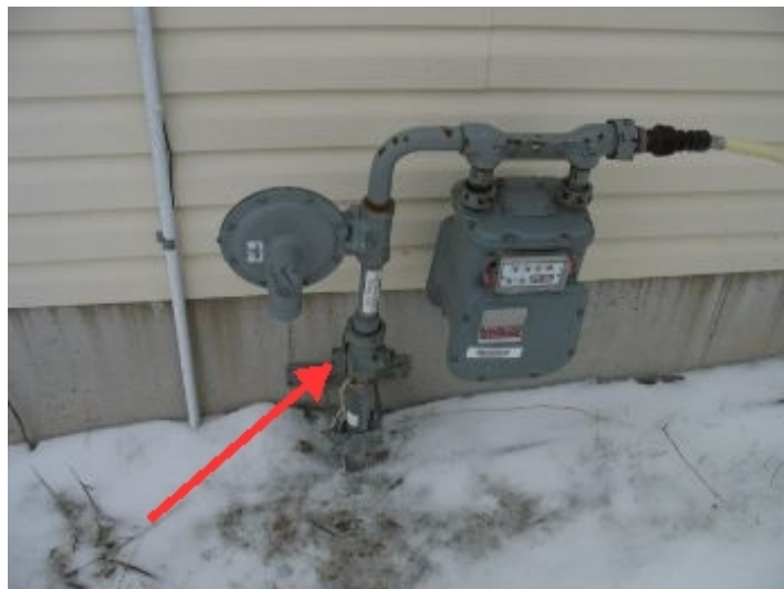
natural gas - main shutoff
