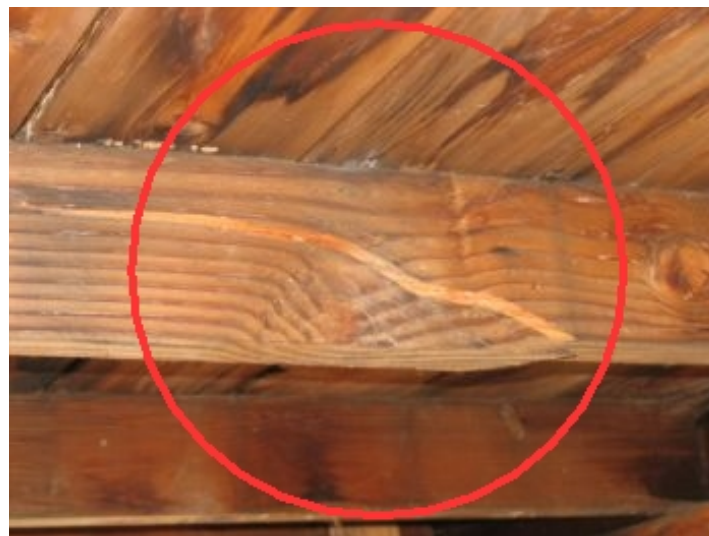
cracked rafters
