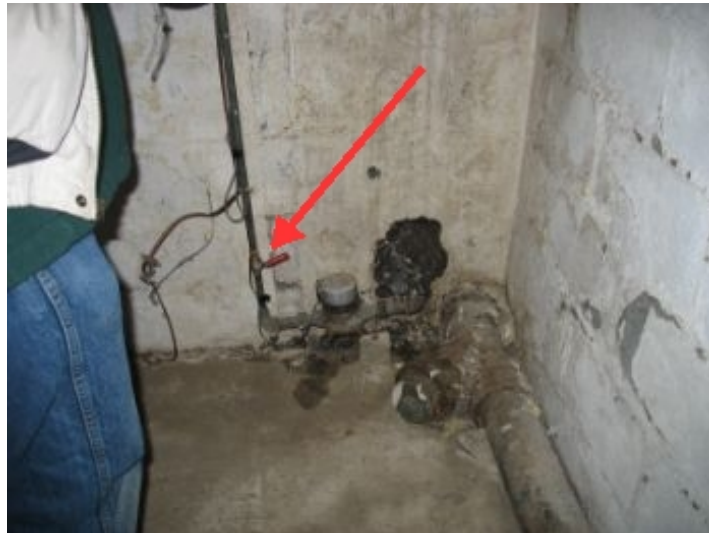
water main shutoff
