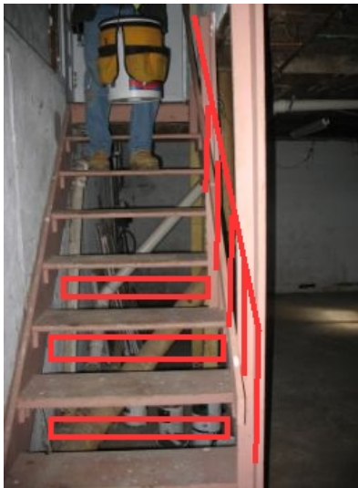
missing handrail / open risers
