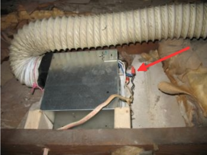
bath fan connection made outside of the housing
