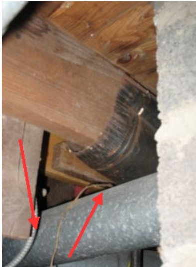
improper clearance to combustible materials
