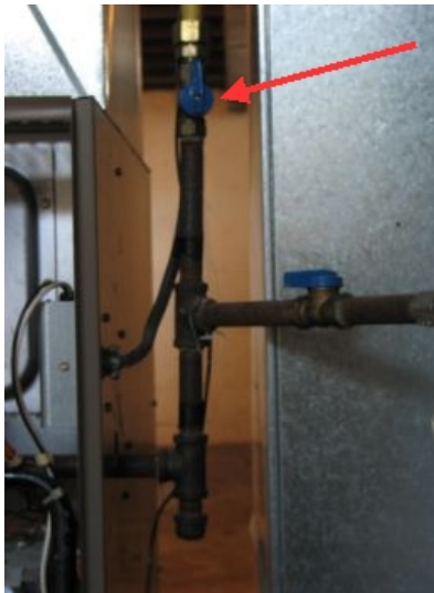
furnace shutoff located to the right 4' up
