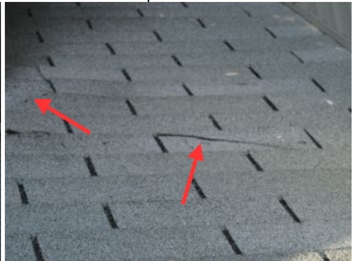
some cracked shingle
